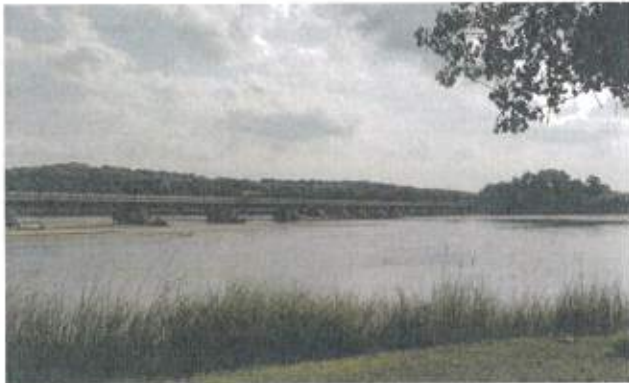
image Lied Platte River Bridge looking southwest
